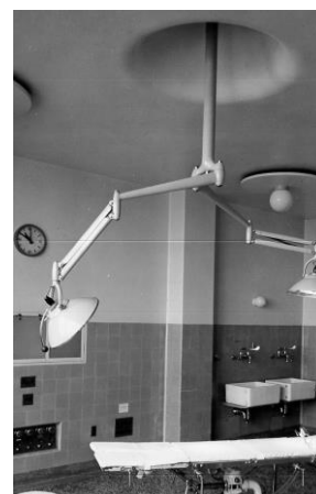
Photo: Theatre Lights
